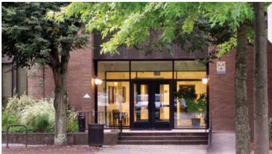
Office of Campus Police Services located in the Administrative Services Building.
